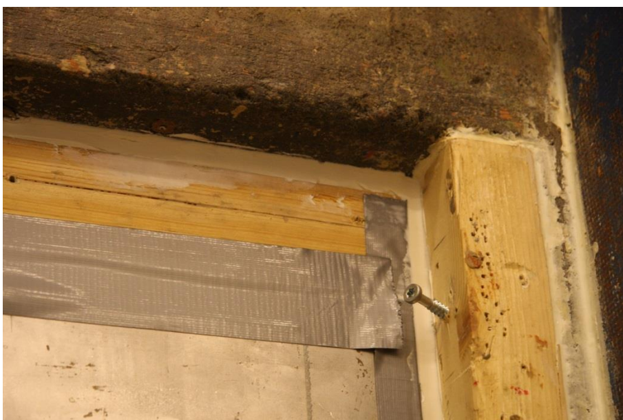
Figure 4 - The sealant applied to the gap.
