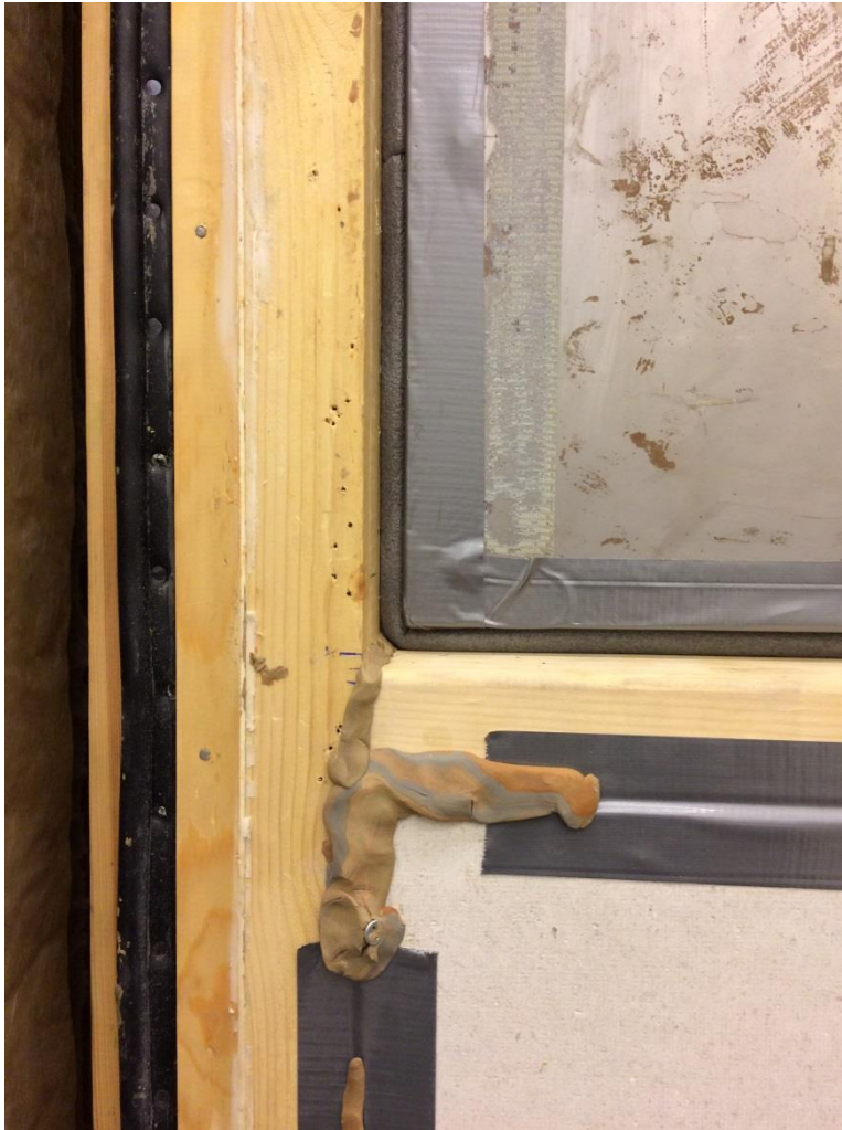
Figure 3 - the backing rod applied to the gap.
